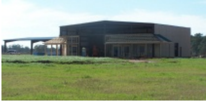
White Oak Pastures nears completion of its new processing plant
